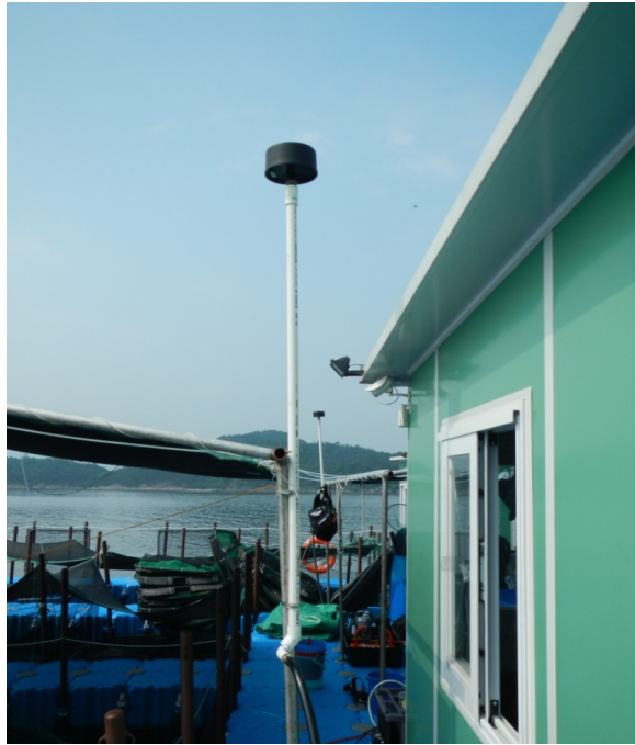
Figure 13. The air inlet filter should be positioned high and away from any machinery exhaust.
